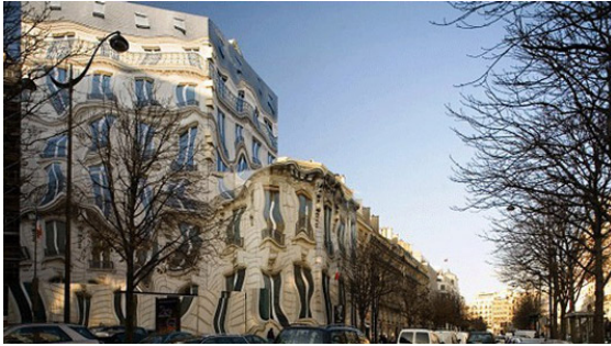
(a) The 39 George V building in Paris.
