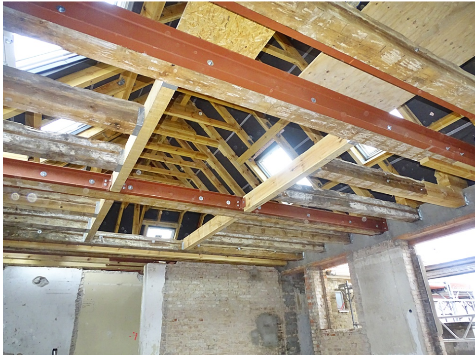
Figure 7. Examined part of the ceiling structure
