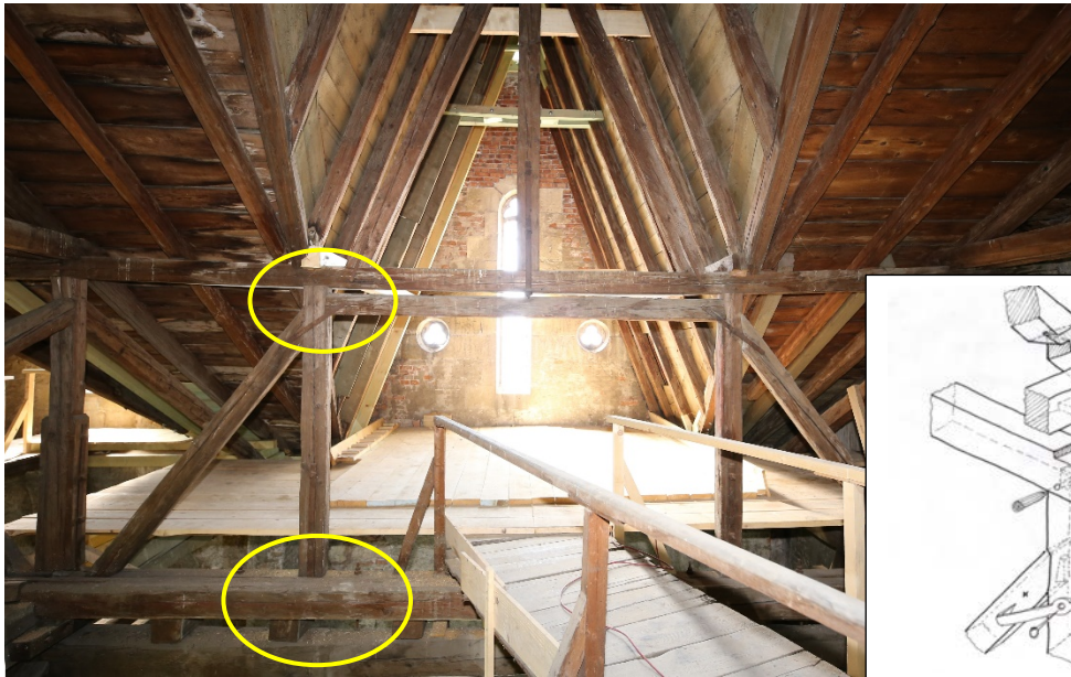
Figure 7 a)-c). Structure above the side aisle of the Zagreb Cathedral (1898). Each of the four segments of the roof with side gable walls spans approximately 6 m. To address this span, the solution involved constructing a beam-like structure, featuring wooden beams as flanges and wooden blocks with through bolts as a web (see lower detail). However, the structure deflected, partly due to the drying of the wood and the pressing of bolt washers into soft firwood, and partly due to the eccentricity of the loading. Additionally, the minimal end-grain surfaces of the queen posts caused compression crushing perpendicular to the fibres of the collar beam (left).
