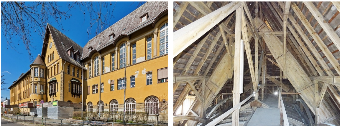
Figure 4. Fichtenberg High School, Berlin/Germany – left: exterior view; right: interior view of the roof construction
