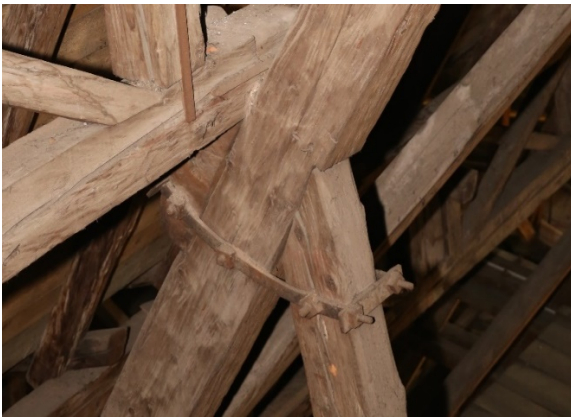
Figure 14 a) and b). Connection detail at the intersection of the principal rafter, main strut, and purlins. The main strut is tenoned approximately 2 cm into the principal rafter and further reinforced by a notched mortise-and-tenon joint to prevent lateral displacement. In the event of structural failure, loosening of the mortise-and-tenon joint would likely precede subsequent displacement, which would be restricted by the cleat and iron stirrup. The cleat and main strut are secured by a robust iron stirrup at the points of compound and I-beam purlin interface. These meticulously executed joints exhibit tight tolerances, high functionality, and exemplary craftsmanship, resulting in reliable structural stability.
