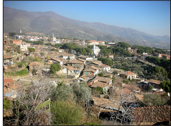
Figure 9. Topographic settlement of the houses in Birgi (Foto: Dışkaya, H.)
