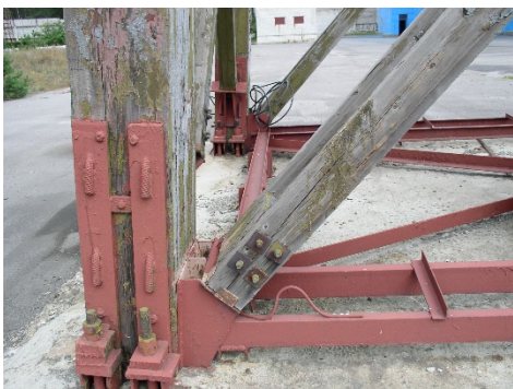
c) support fastening on inclined glued-in rods) examination 2011 (Prof. Fursov and PhD-student Bidakov)
