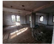
Photo 4 – Second floor of the extension
