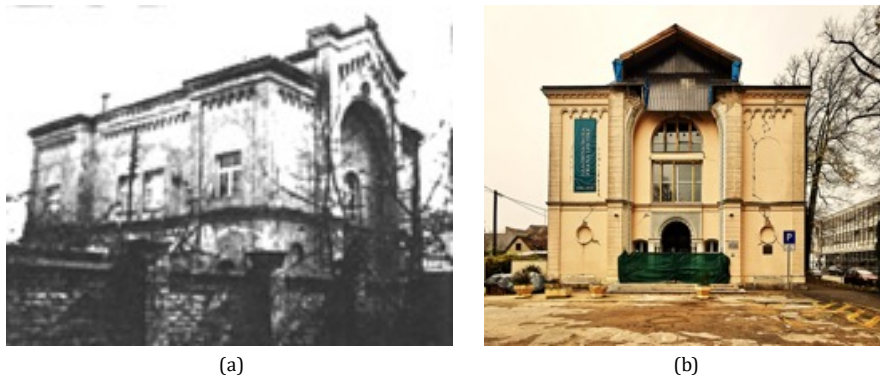
Figure 1. Building before the earthquake (a) and its front western façade after the 2020 earthquake (b).
