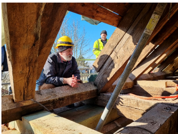
Figure 21. The work of an expert on-site consists of careful observations, crawling on the floor, and hanging from the trusses (the structural framework that supports the roof). The expert approaches the object with a camera and light, as well as measurement tools and scientific instruments used to assess its structural integrity. The process concludes with a discussion among all the involved parties, including carpenters, to achieve a satisfactory outcome for all. Photo by J. Pojatina.
