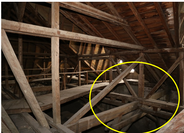
Figure 19 a) and b). Connections of the principal rafters to the king post at the ridge. Various solutions were found. The option seen in the photograph and the left sketch used housed notched joints with mortise and tenon. These were secured either by stirrups or by clamps with a central bolt. The solution on the right, a simple notched joint with clamps, was not firm enough and opened over time.
