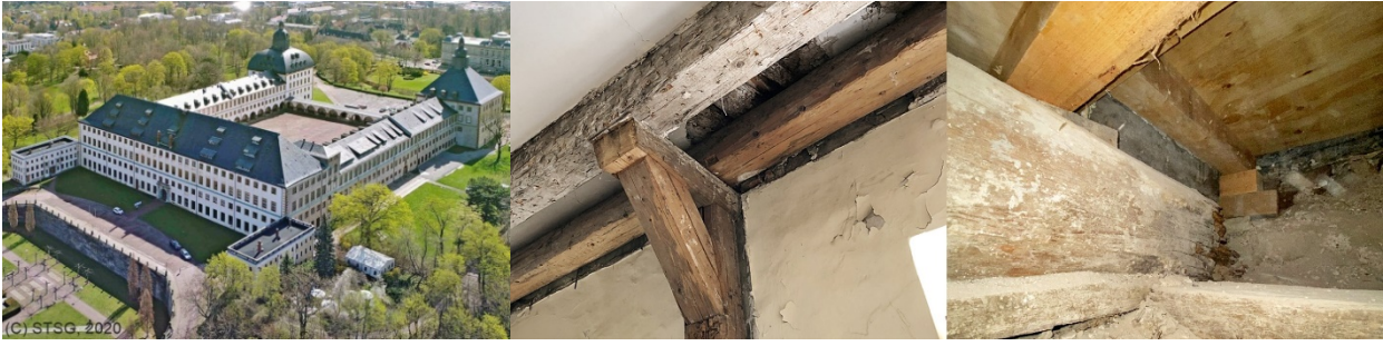
Figure 5. Castel Friedenstein, Gotha/Germany – left: aerial view; right: examined ceiling construction
