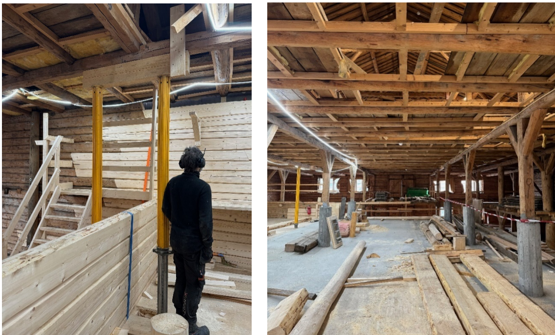
Figure 2. Brygge 15 during adaptation: replacement of rotten timber (left), concrete structure from the 1980s.
