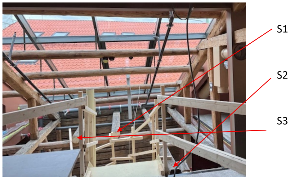
Figure 4. Specimens S1, S2, S3 measured in situ after adaptation (renovation), Brygge 15, Trondheim
