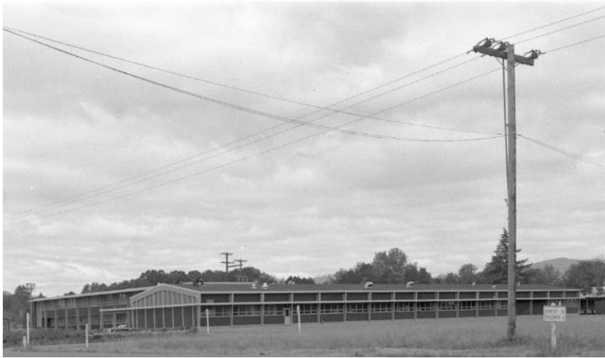
Figure 32. The Oregon Forest Research Laboratory (later renamed the Oak Creek Building), captured soon after completion in 1956 [17], showing a sunshade circumnavigating the perimeter of the building.
