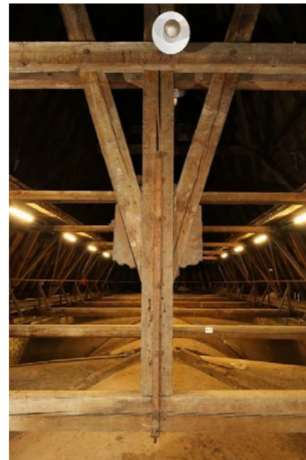
Figure 16 a)–c). Notable deviation from conventional engineering practice. The tie beams exhibit inverse deflection (left). Rather than maintaining a gap between the king post and tie beams, the beams are fitted with stirrups that induce upward tension toward the post (middle). Consequently, the entire truss assembly is tensioned, initiating at the tie beams and subsequently tightening each truss joint in progression.
