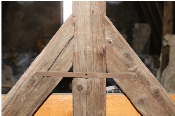
Figure 19 a) and b). Connections of the principal rafters to the king post at the ridge. Various solutions were found. The option seen in the photograph and the left sketch used housed notched joints with mortise and tenon. These were secured either by stirrups or by clamps with a central bolt. The solution on the right, a simple notched joint with clamps, was not firm enough and opened over time.
