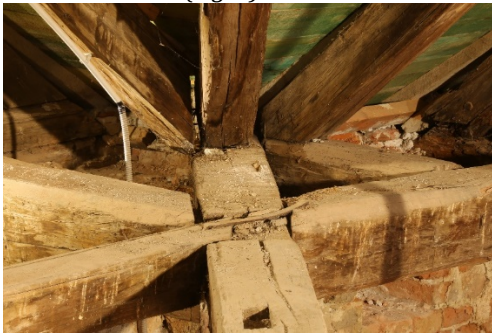
Figure 3 a) and b). The joints in the perimeter grid are positioned inadequately. Failure results when the lap joint and tenon coincide in plane, causing wood to fail in shear and tension perpendicular to fibres.
