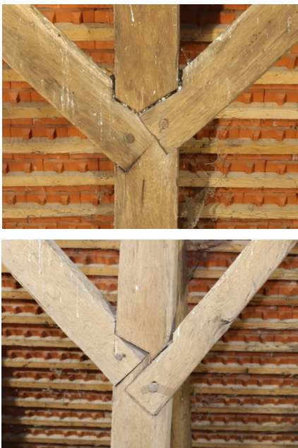
Figure 4 a)-c). Church of St. Michael Archangel, Prelošćica, 1832. Shown here are examples of curiously misshapen blind dovetail laps of knee brackets. The structural problems are as follows: depending on the load, the wood fails in compression perpendicular to fibres (compression) or splits in shear or tension perpendicular to fibres (tension). Additionally, positioning wooden pegs too close to the edge of the post can cause the post to split along its grain. These issues suggest that the church was presumably built by local carpenters with limited experience in carpentry.
