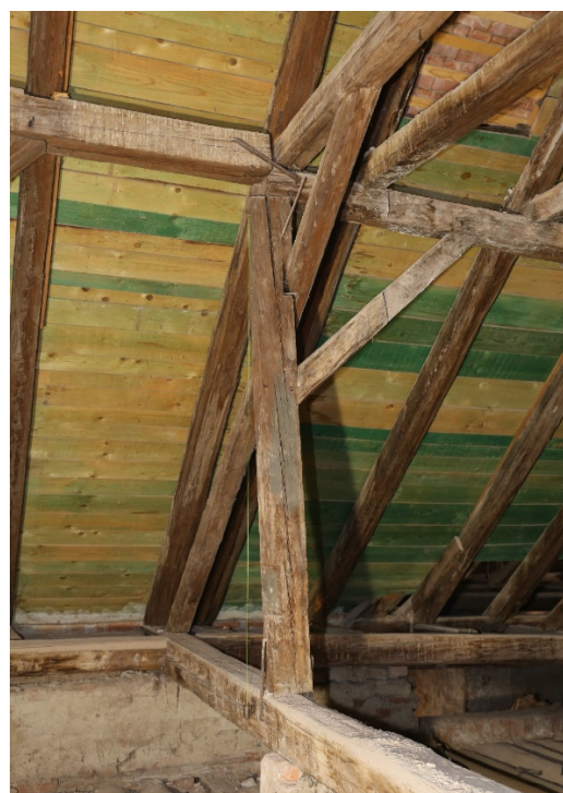
Figure 1 a)-c). Upper Town High School (origin of the Zagreb University, 1695). The sequence of failures begins with inadequately chosen joints: the strut is too shallowly lapped on the post without a dowel, there is a too-small dovetail lap with the collar, and the collar does not adequately "catch" the purlin on top of the post. These lead first to shear failures at the upper left dovetail lap joint, followed by rotation of the post due to shear failure in the collar. As the collar tie fails, a crack forms in the post, and the post inclines outward (upper left). The lower sketch shows the incorrect layout of the rafter on the collar, which subsequently fails in shear. The right sketch presents a better solution for queen-post structures. Red lines indicate possible remedial measures. Iron clamps are not sufficiently strong and secure for binding the elements, particularly not in softwoods.
