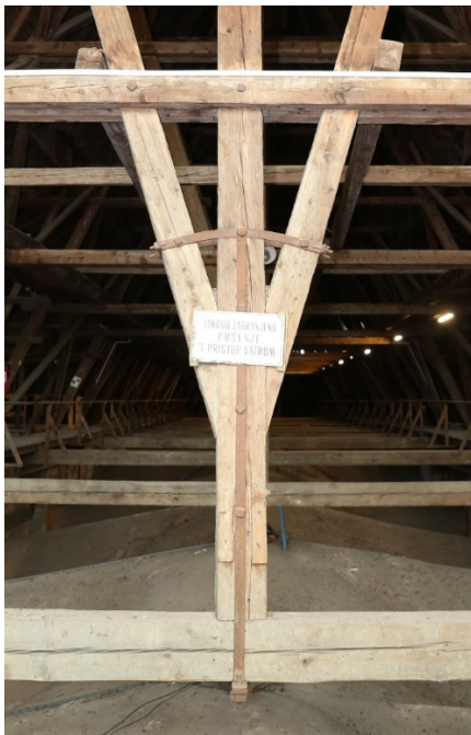
Figure 16 a)–c). Notable deviation from conventional engineering practice. The tie beams exhibit inverse deflection (left). Rather than maintaining a gap between the king post and tie beams, the beams are fitted with stirrups that induce upward tension toward the post (middle). Consequently, the entire truss assembly is tensioned, initiating at the tie beams and subsequently tightening each truss joint in progression.
