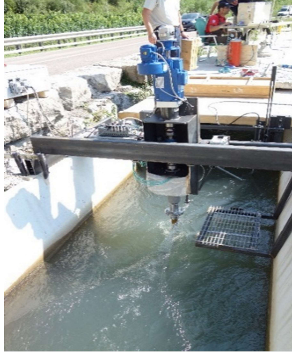
Fig. 1-1. The hydrokinetic turbine and its structural support mounted on the embankments.
