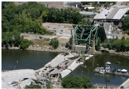
Figure 2.4: Progressive collapse of the Mississippi River Bridge
