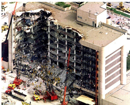
Figure 2.5: Progressive collapse of the Murrah Federal Building
