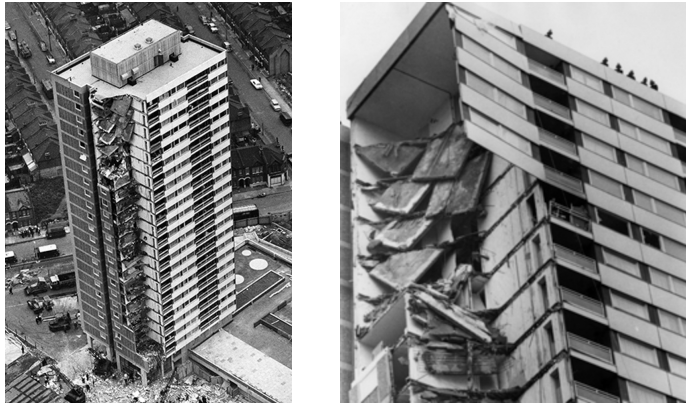
Figure 2.6: Progressive collapse of Ronan Point Building
