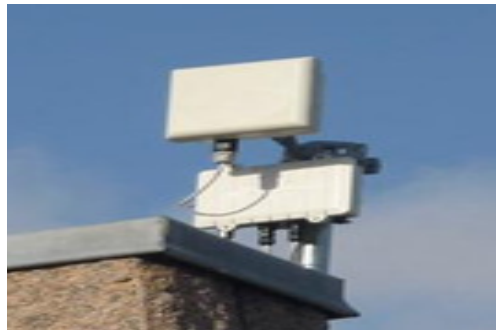
(b) Outdoor Base Station
