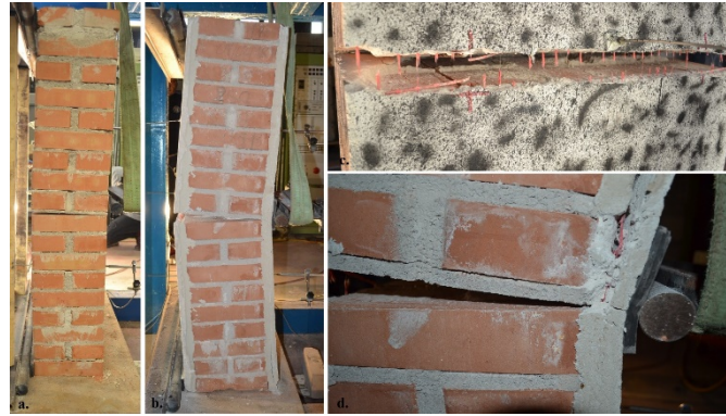
Fig. 17 – Failure modes of the unstrengthened (a) and strengthened (b,c,d) fired clay brick masonry walls.
