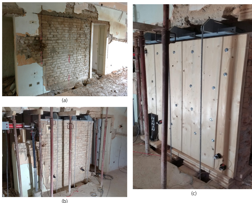
Figure 3. Specimen preparation: (a) specimen after removal of plaster and creation of through cuts; (b) specimen AsB-1 prior to testing; (c) specimen R-1 prior to testing
