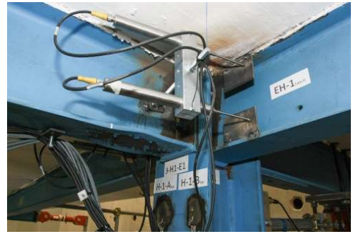
(b) Buckling of the beam flange at joint G
