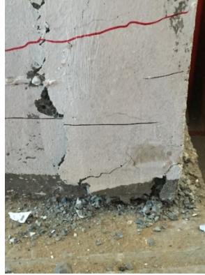
(a) Bottom of the pier in the left side
