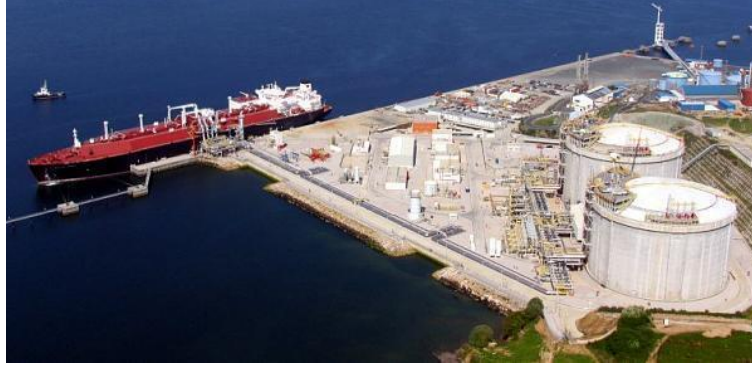
Fig. 1. Refrigerated liquefied gas plant overview
